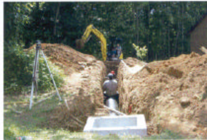
Drop Inlet Construction
