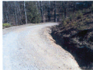
Eroding Ditch
